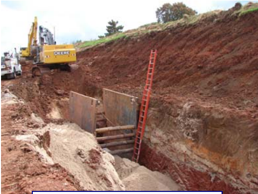
Nick Taylor and Mike Anderson Laying Pipe in Oklahoma City
